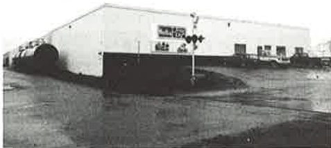
Hostess Frito-Lay, New Minas, N.S. ($85,000 in tax savings)
