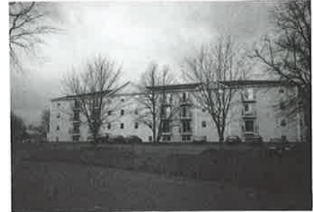
Kensington Road, Charlottetown, P.E.I. ($9,000/annum - 24% in tax savings)
