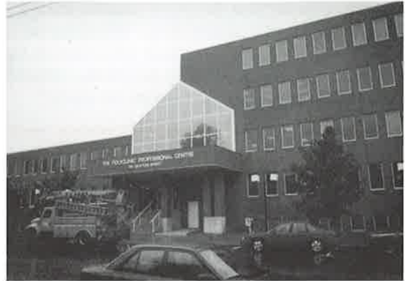
Polyclinic, Charlottetown, P.E.I. ($22,000/annum - 12% in tax savings)
