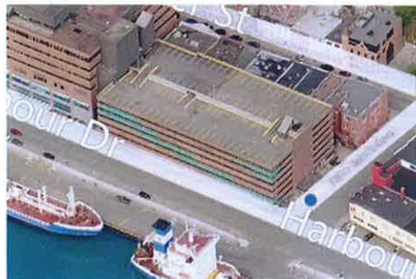
Parking Garage, Newfoundland ($199,119 - 23% in tax savings)
