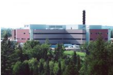
Upper River Valley Hospital, Waterville, N.B.
